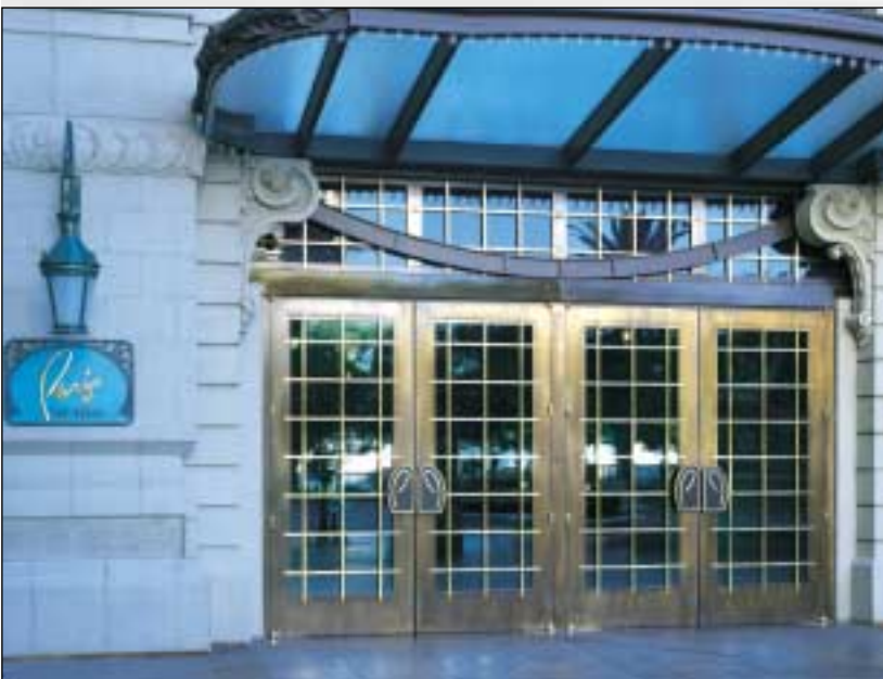
Paris Hotel & Casino, Las Vegas, Nevada Architect: Bergman-Walls & Youngblood also the Hilton Corporation
